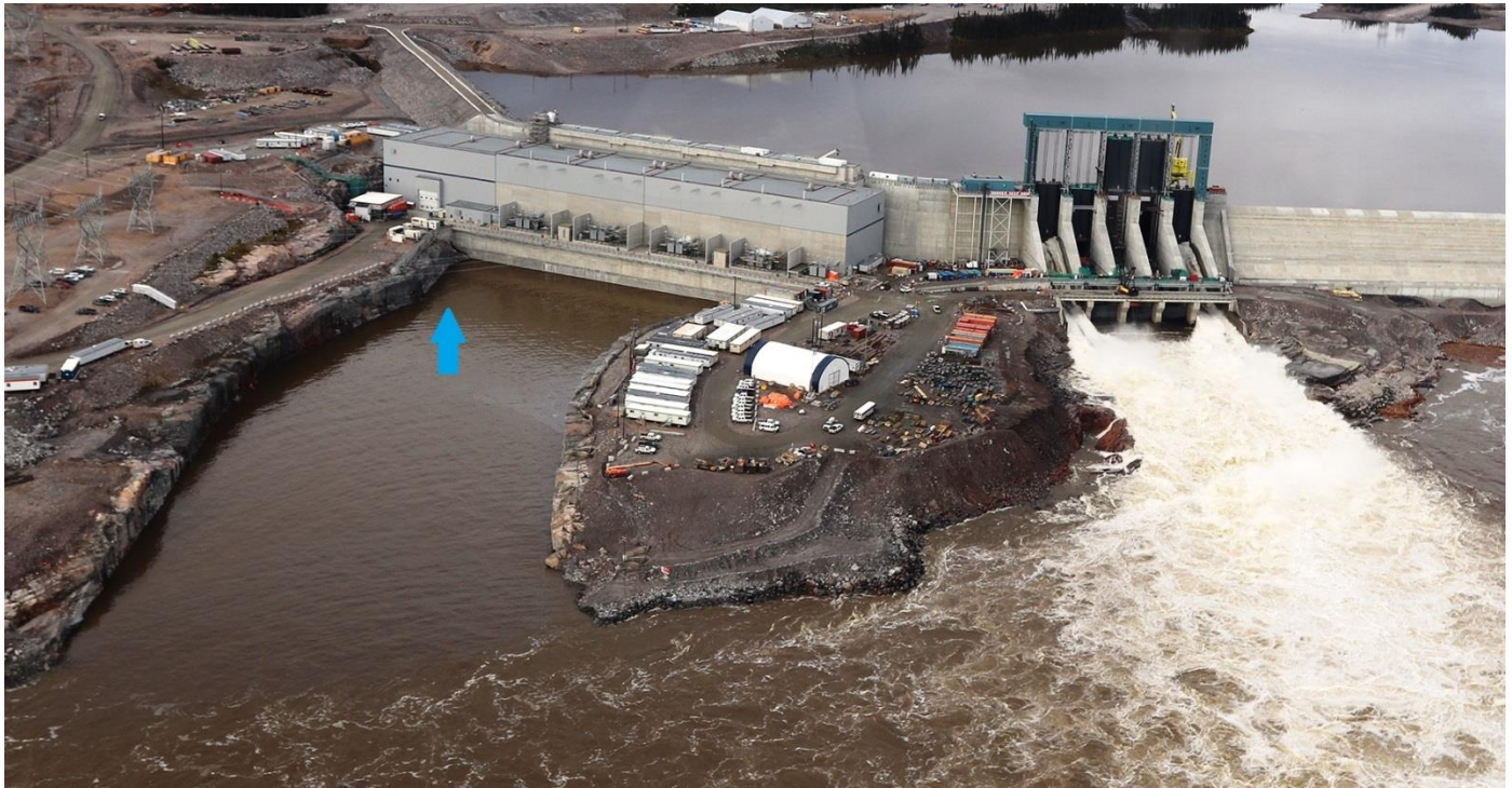
Caption: Tailrace channel with location of oil sheen
