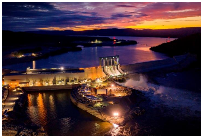
Muskrat Falls generating facility at night
