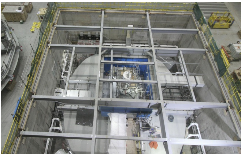
Muskrat Falls Powerhouse – overlooking work on Unit #2
