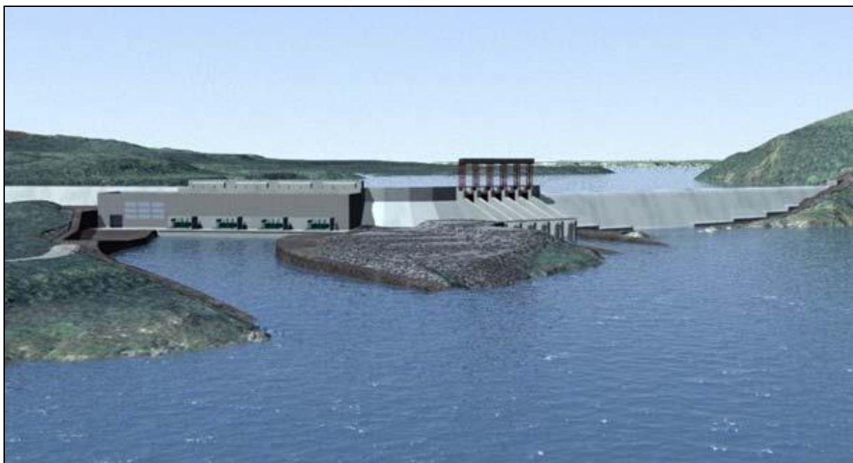
Figure 5-1 Muskrat Falls Generating Facility
