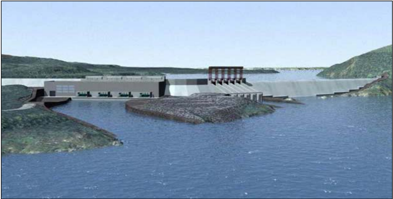
Figure 5-1 Muskrat Falls Generating Facility
