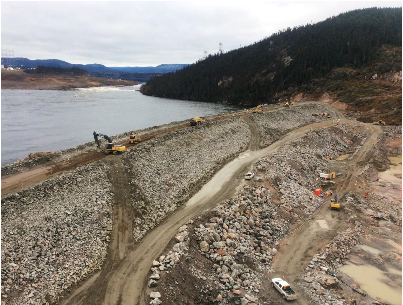
Figure 8-2 Photo of the Temporary Cofferdam Constructed at Muskrat Falls, November 2016
