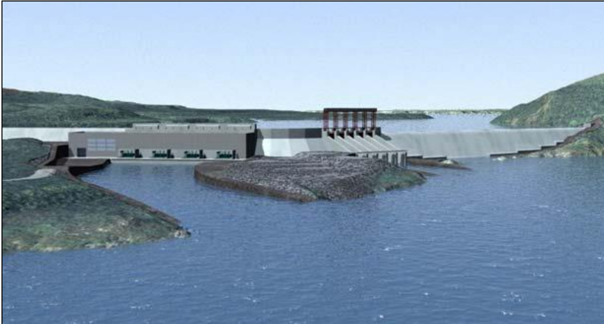
Figure 7-1 Muskrat Falls Generating Facility
