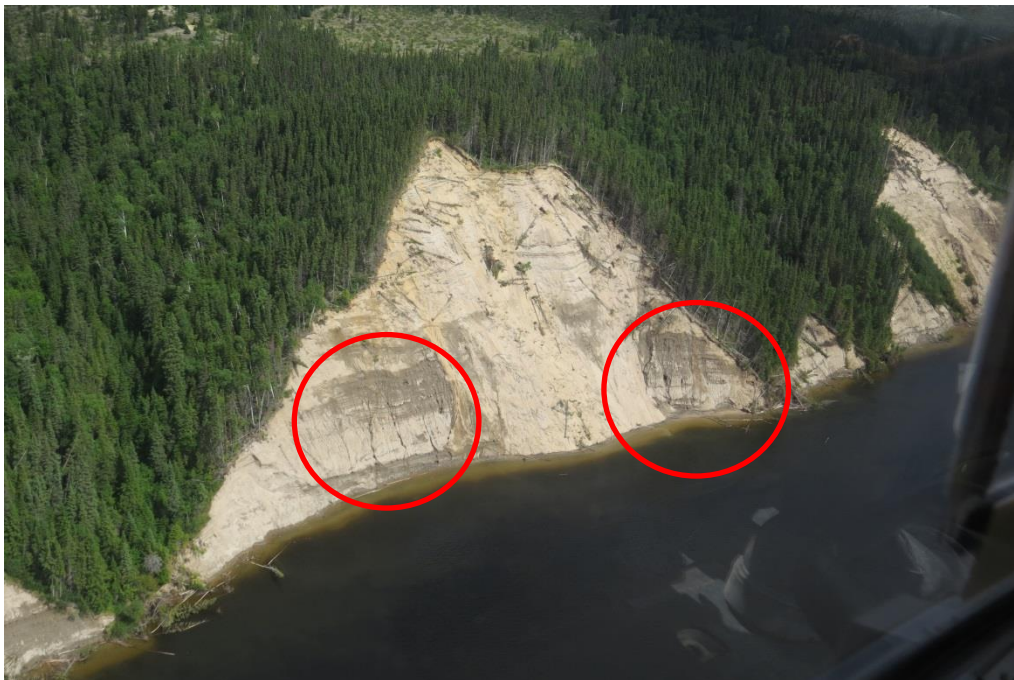
Figure 3: Kilometer 48 North Bank, active erosion
