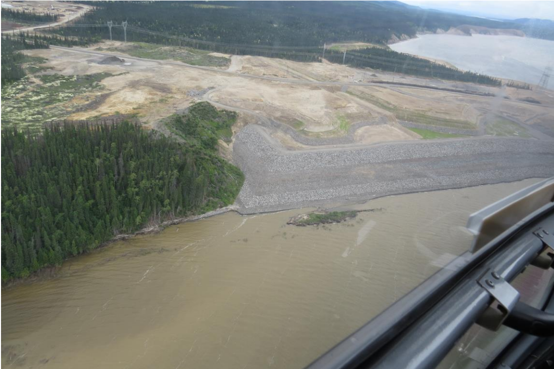
Figure 4: North Bank 45 km, Heavy sedimentation
