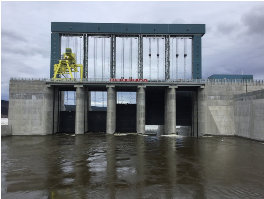
Upstream side of the spillway on May 19, 2017. Gates 1 & 2 are open; and Gates 3, 4 & 5 are partially open. Gates are numbered 1 to 5 from right to left.
