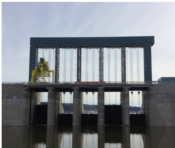
Upstream side of the spillway on April 28, 2017. Gates 1, 3 & 4 are closed; and Gates 2 & 5 are partially open. Gates are numbered 1 to 5 from right to left.
