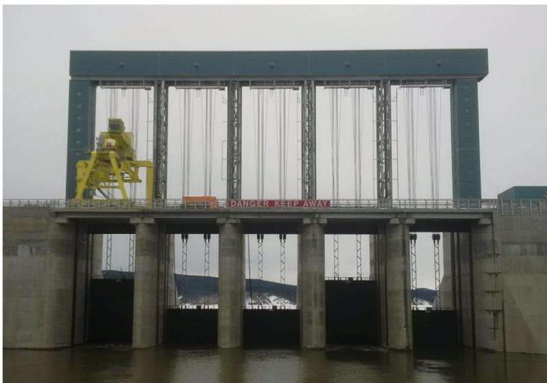
*Upstream side of the spillway on April 13, 2017. Gates 1, 3 & 4 are closed; and Gates 2 & 5 are partially open. Gates are numbered 1 to 5 from right to left.*
