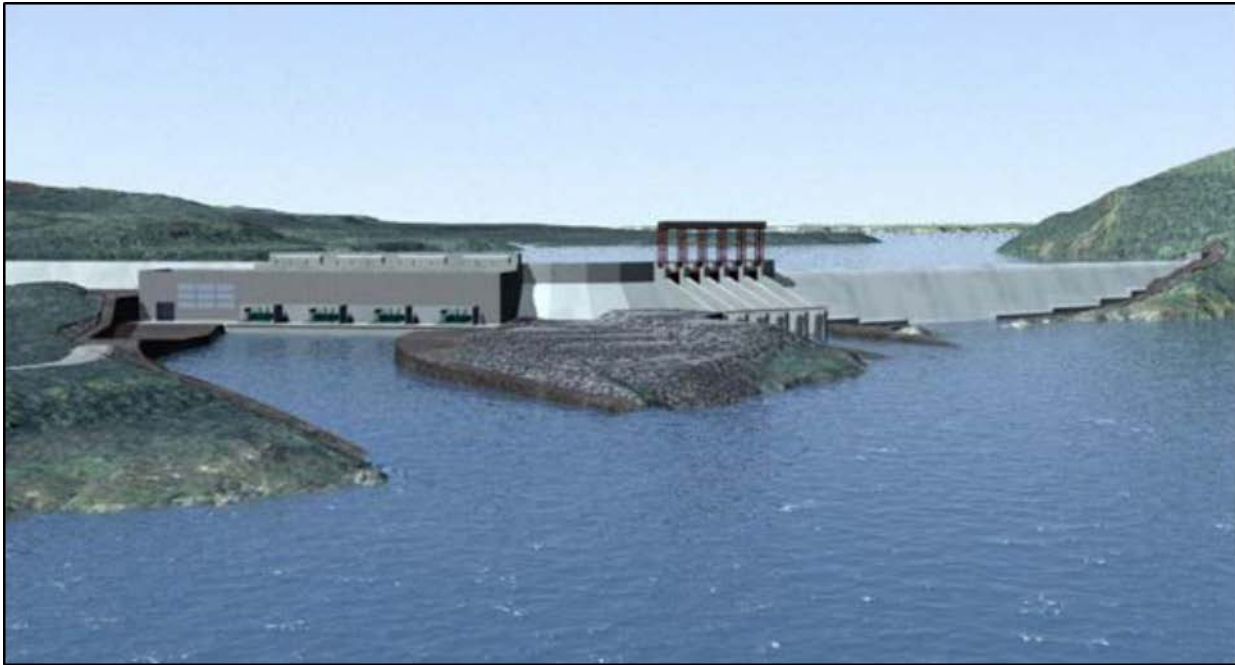
Figure 6-1 Muskrat Falls Generating Facility
