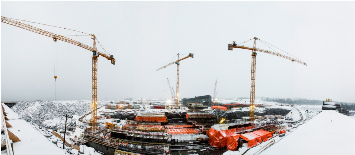
Construction work by Astaldi Canada on the spillway for Muskrat Falls.
