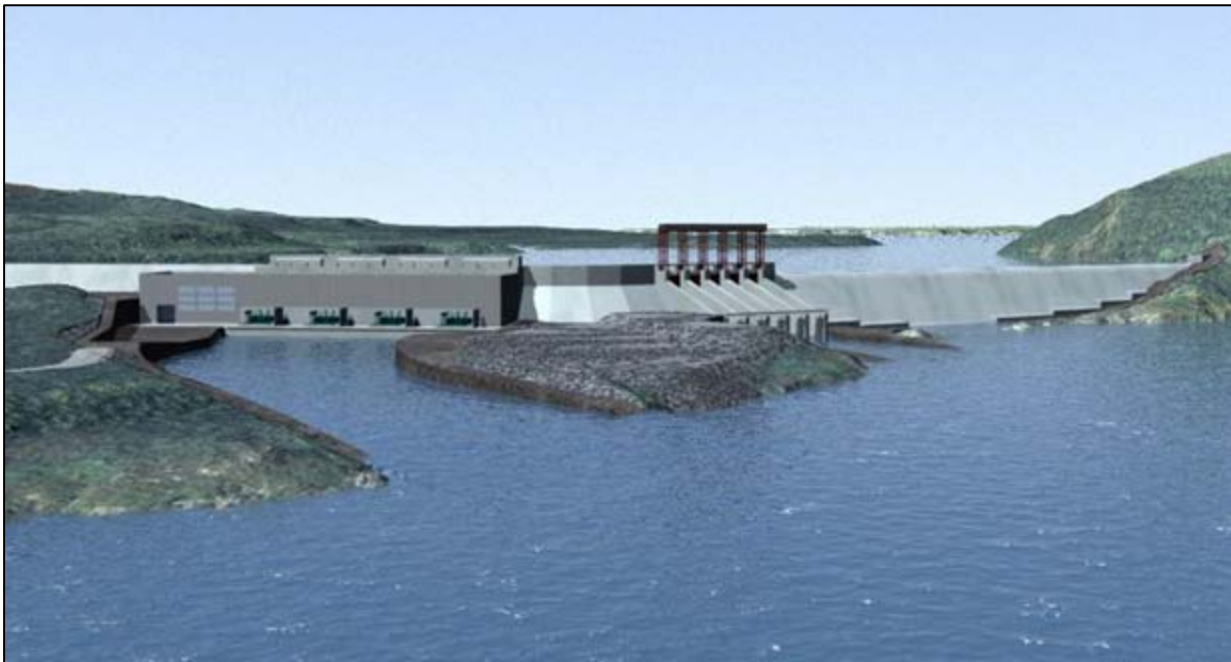
Figure 6-1 Muskrat Falls Generating Facility
