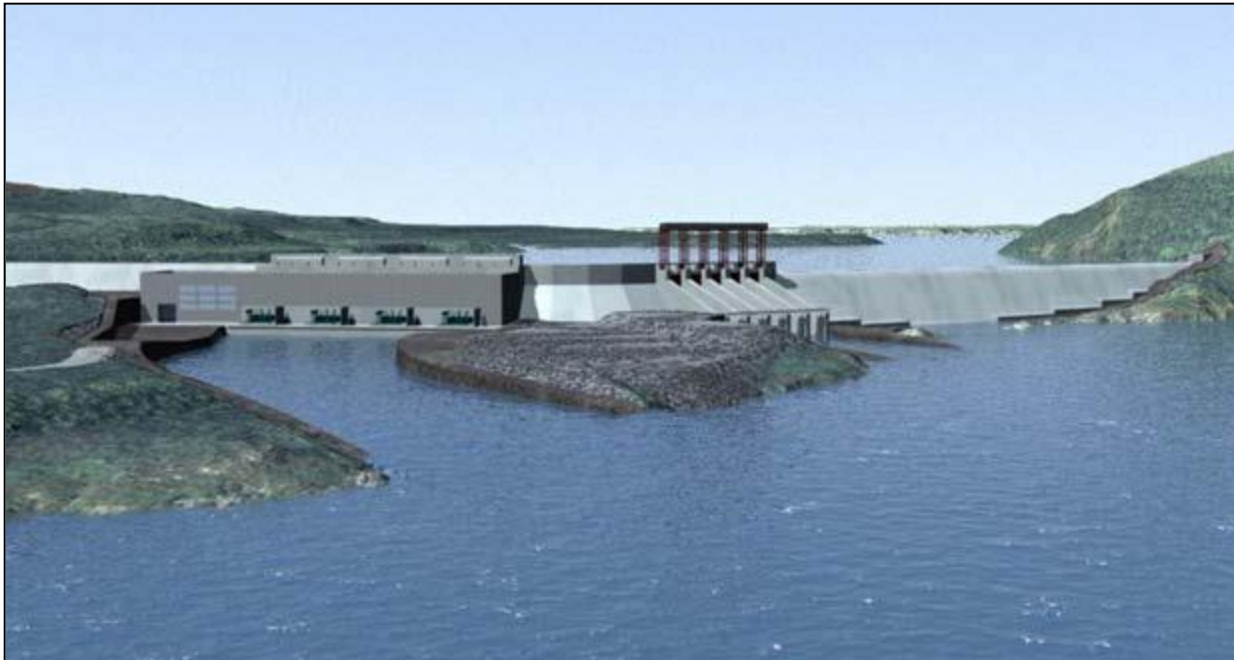
Figure 6-1 Muskrat Falls Generating Facility
