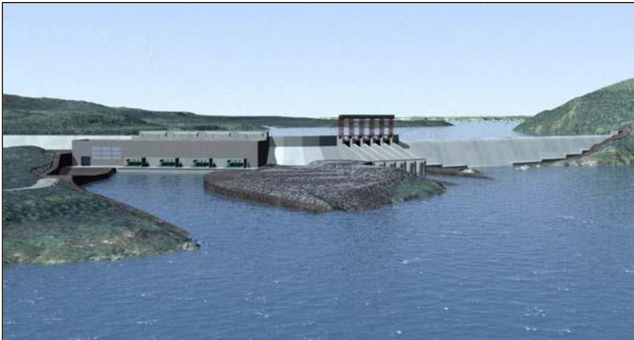
Figure 4-1 Muskrat Falls Generating Facility
