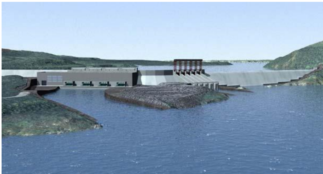
Figure 6-1: Muskrat Falls Generating Facility
