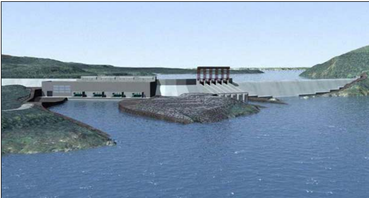
Figure 5-1 Muskrat Falls Generating Facility
