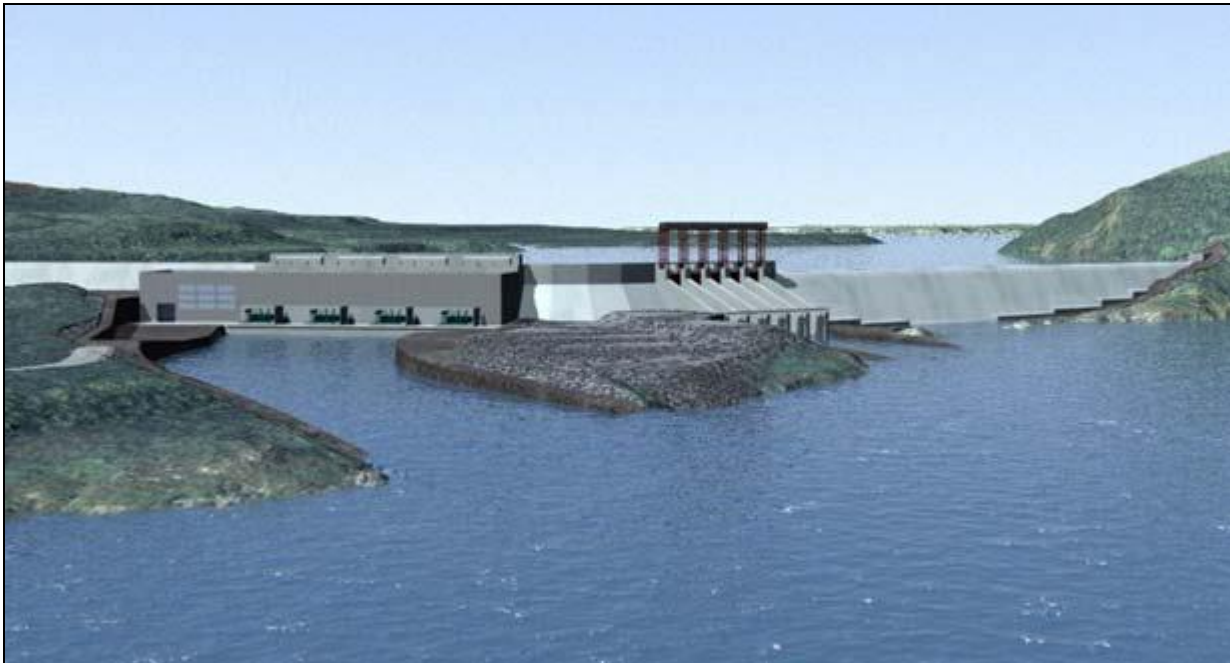
Figure 11-1 Muskrat Falls Generating Facility
