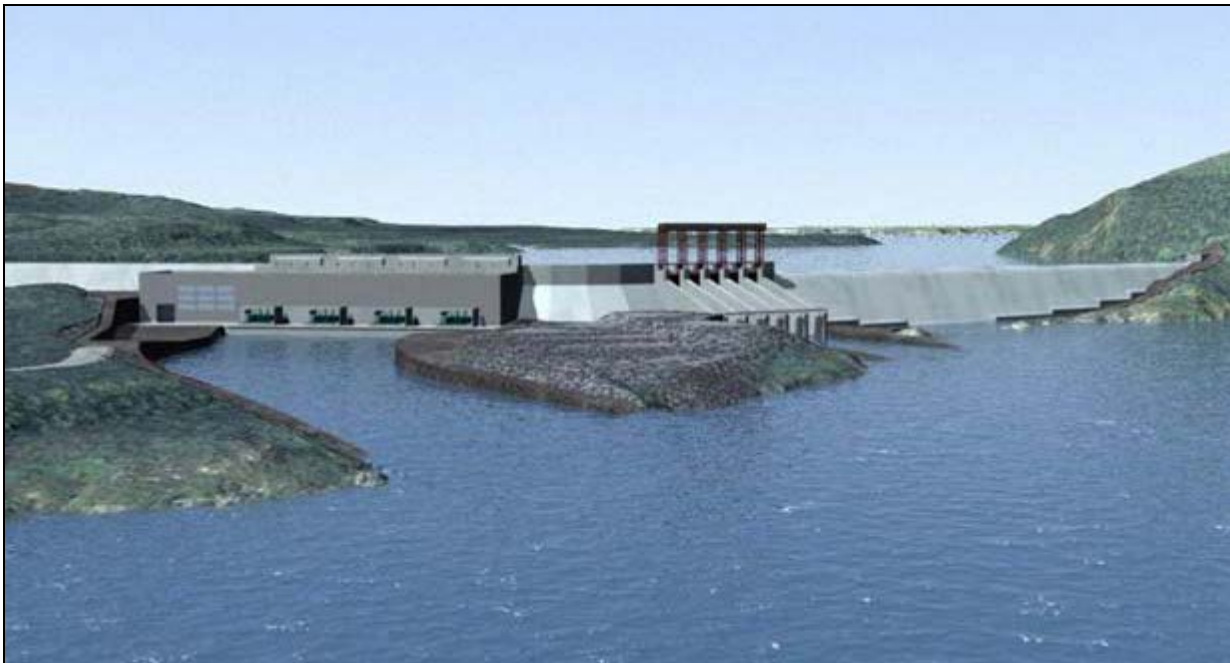
Figure 5-1 Muskrat Falls Generating Facility
