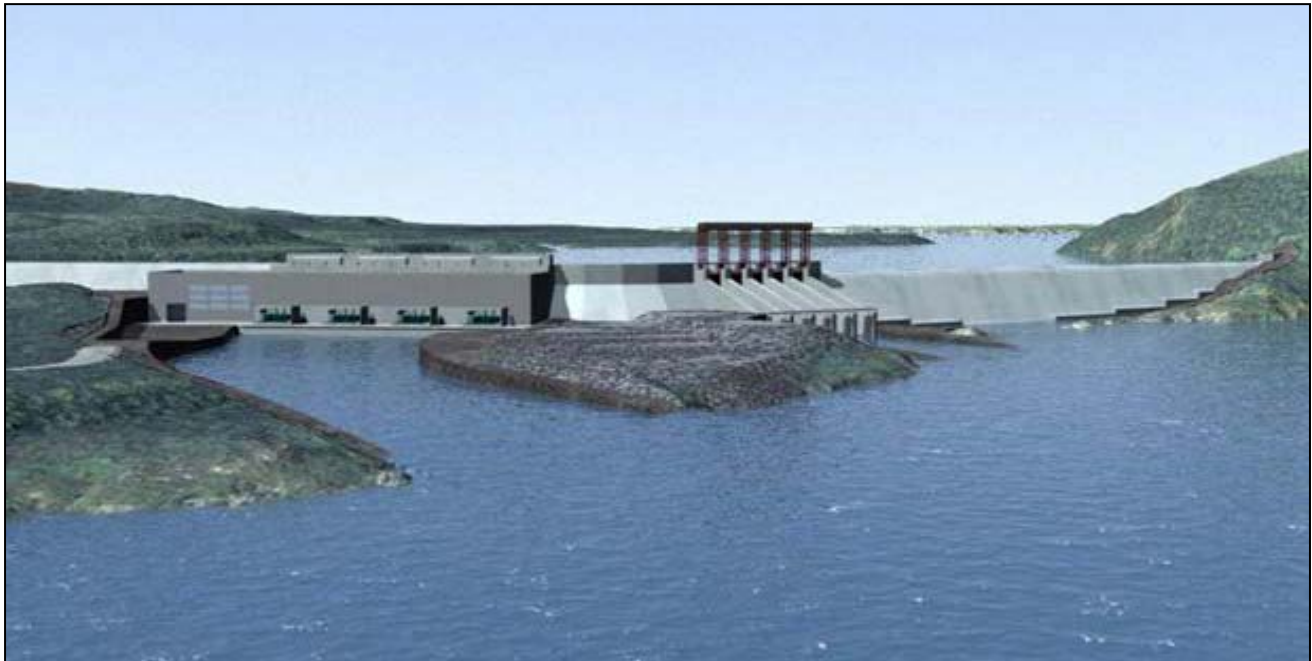
Figure 6-1 Muskrat Falls Generating Facility
