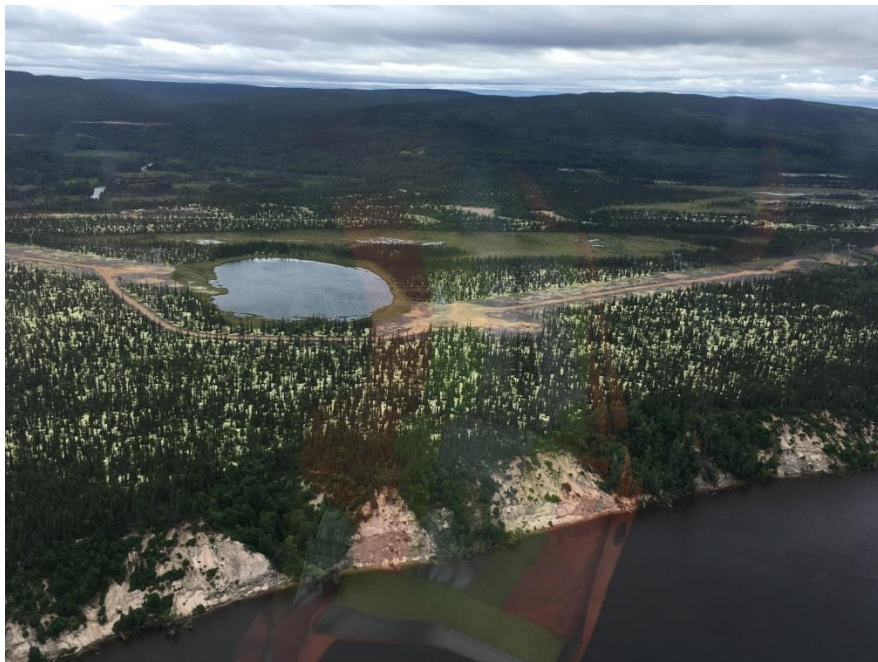
Slope at KM 49 with pond and tower line in upstream.
