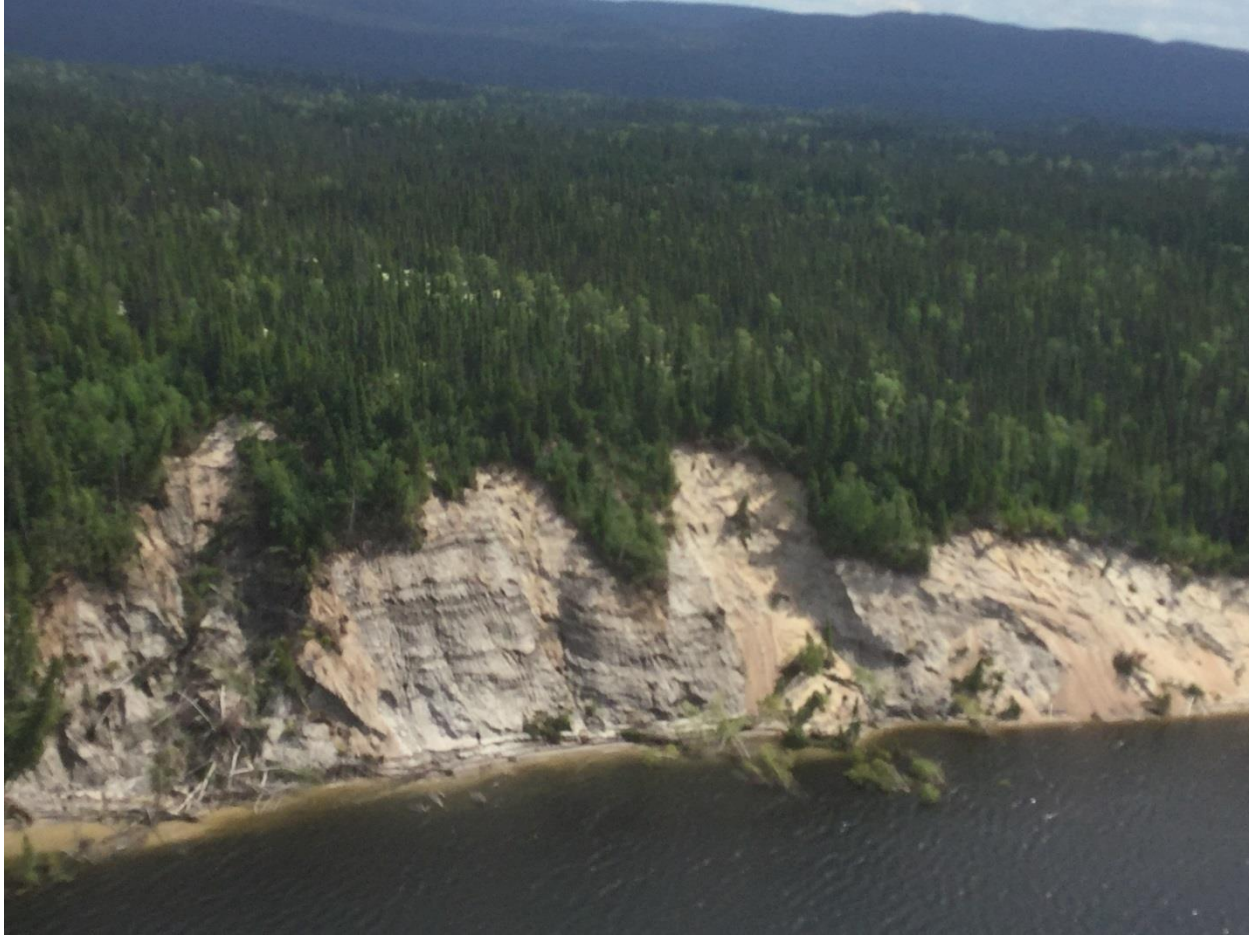
Figure 3: Some erosion between 67 and 68 Km South Bank
