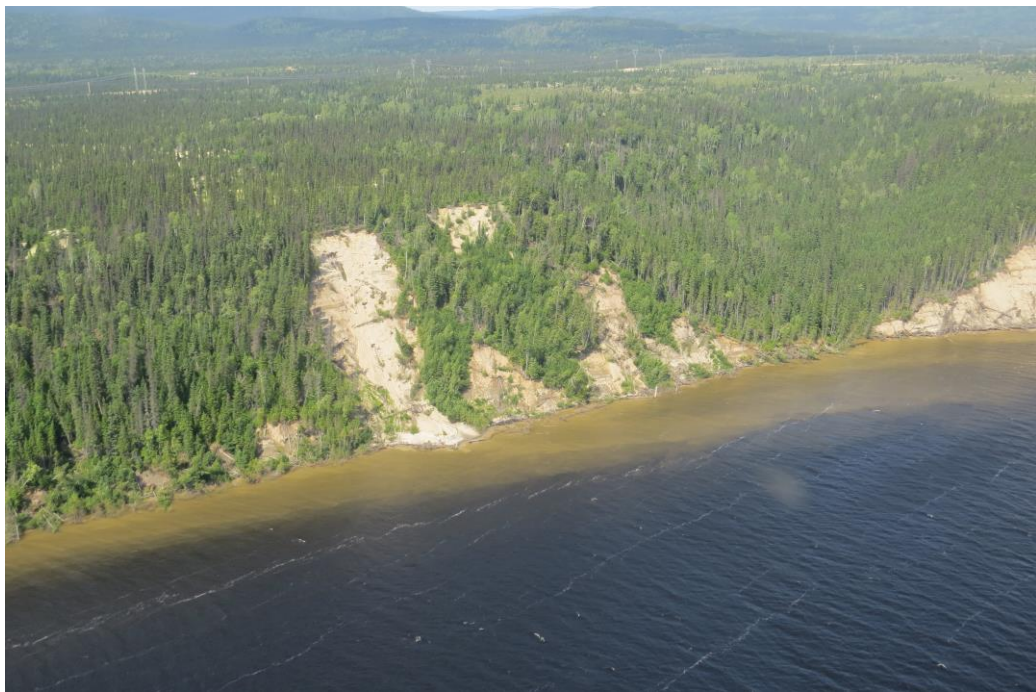
Figure 3: About 78 km, Left Bank
