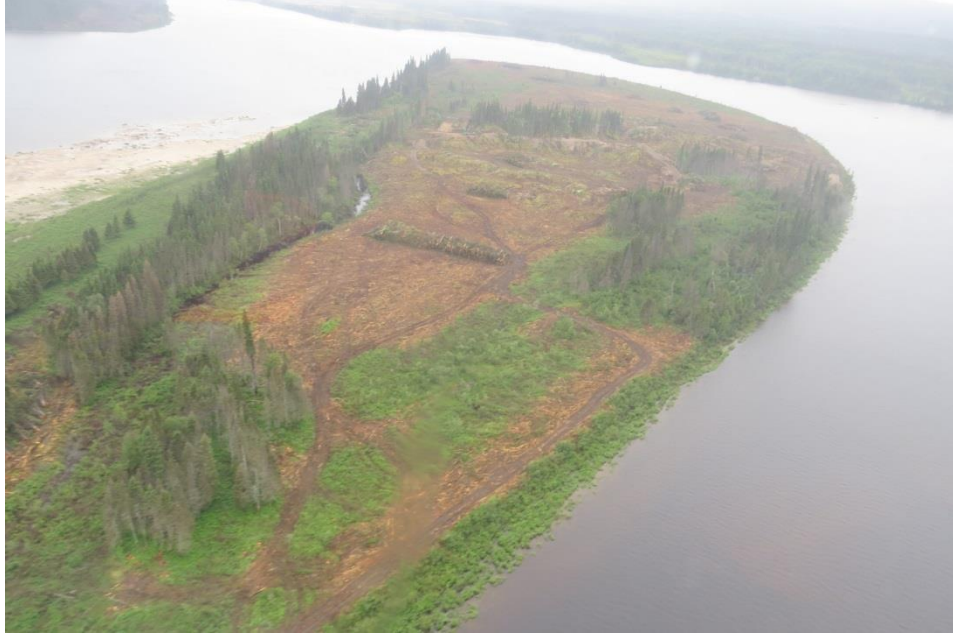
Figure 2: Edwards Island being cleared
