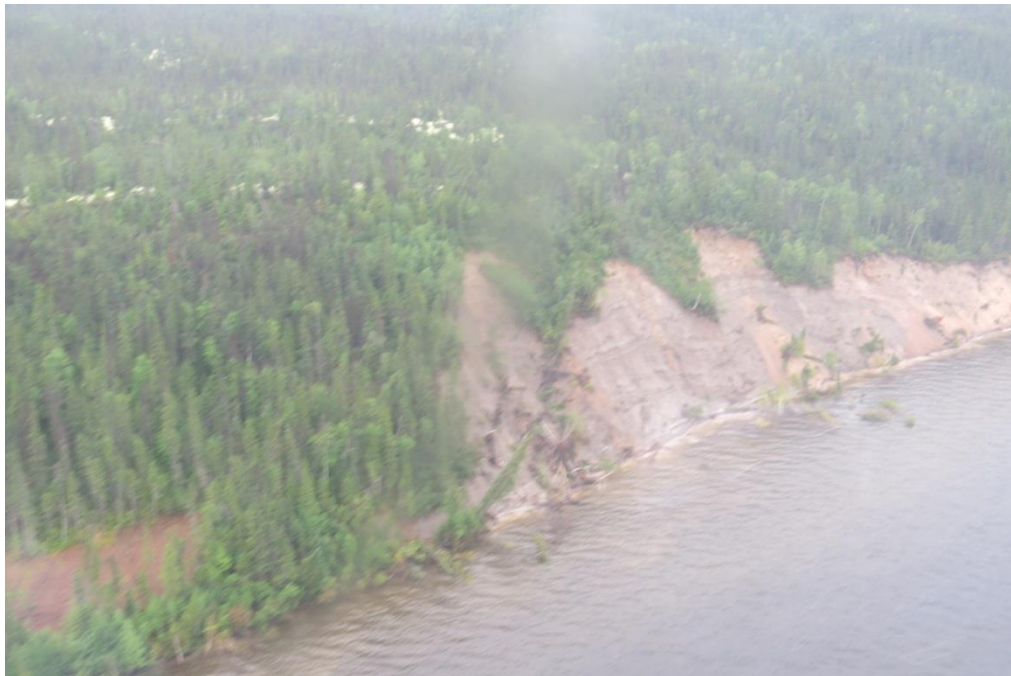
Figure 1: Between 67 to 68 Km, South Bank
