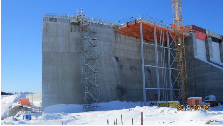
Centre transition dam
