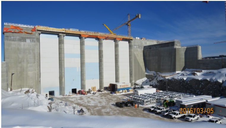
Upstream view of the spillway piers
