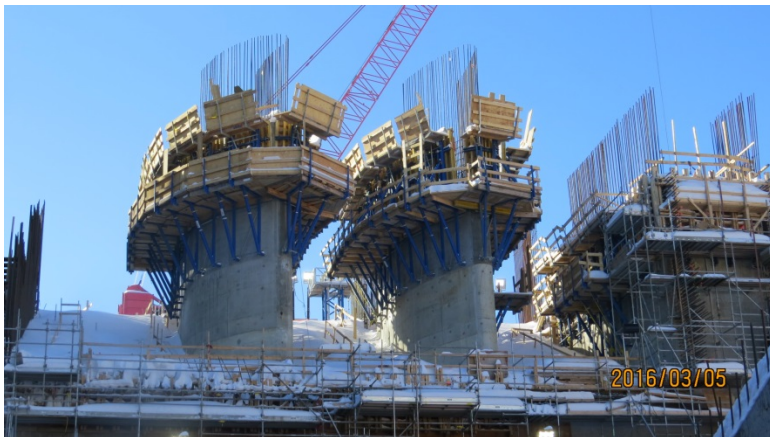
Downstream view of the intake
