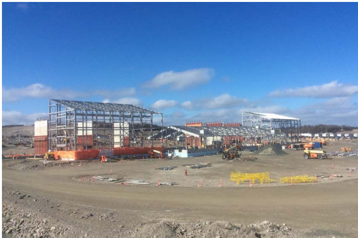
Control building for the Soldiers Pond converter station Stringing conductor wire on the transmission line from Muskrat Falls to Churchill Falls
