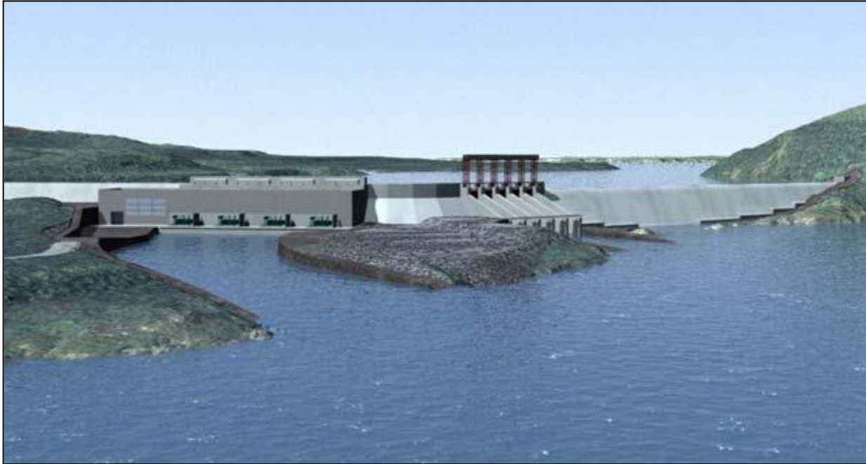
Figure 6-1 Muskrat Falls Generating Facility
