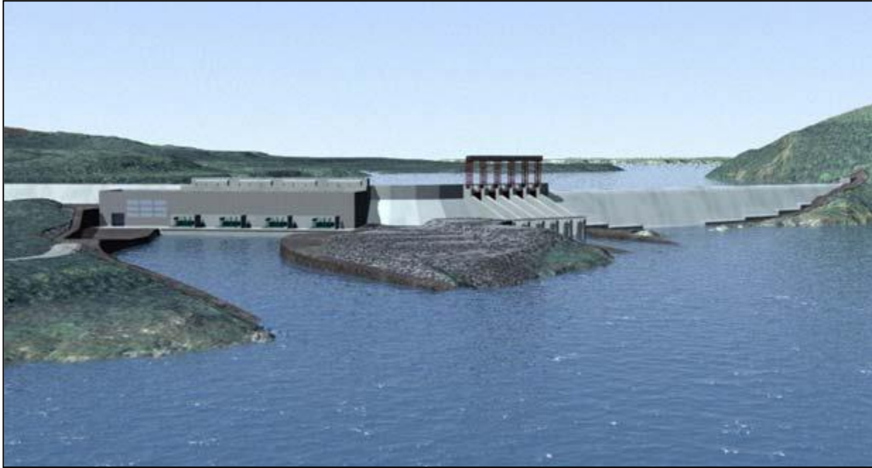
Figure 6-1 Muskrat Falls Generating Facility
